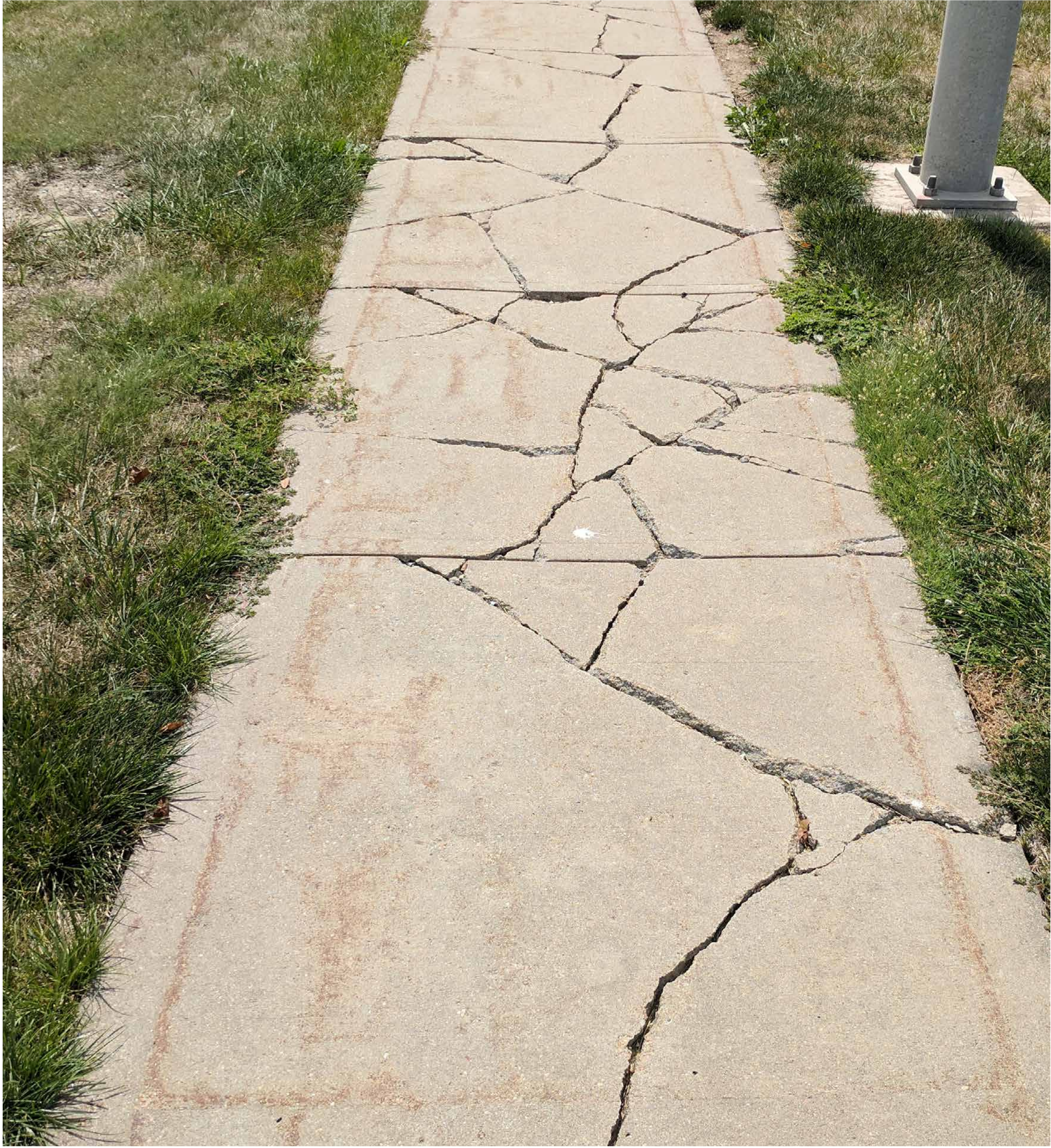
Existing 4' detached sidewalk in poor condition
