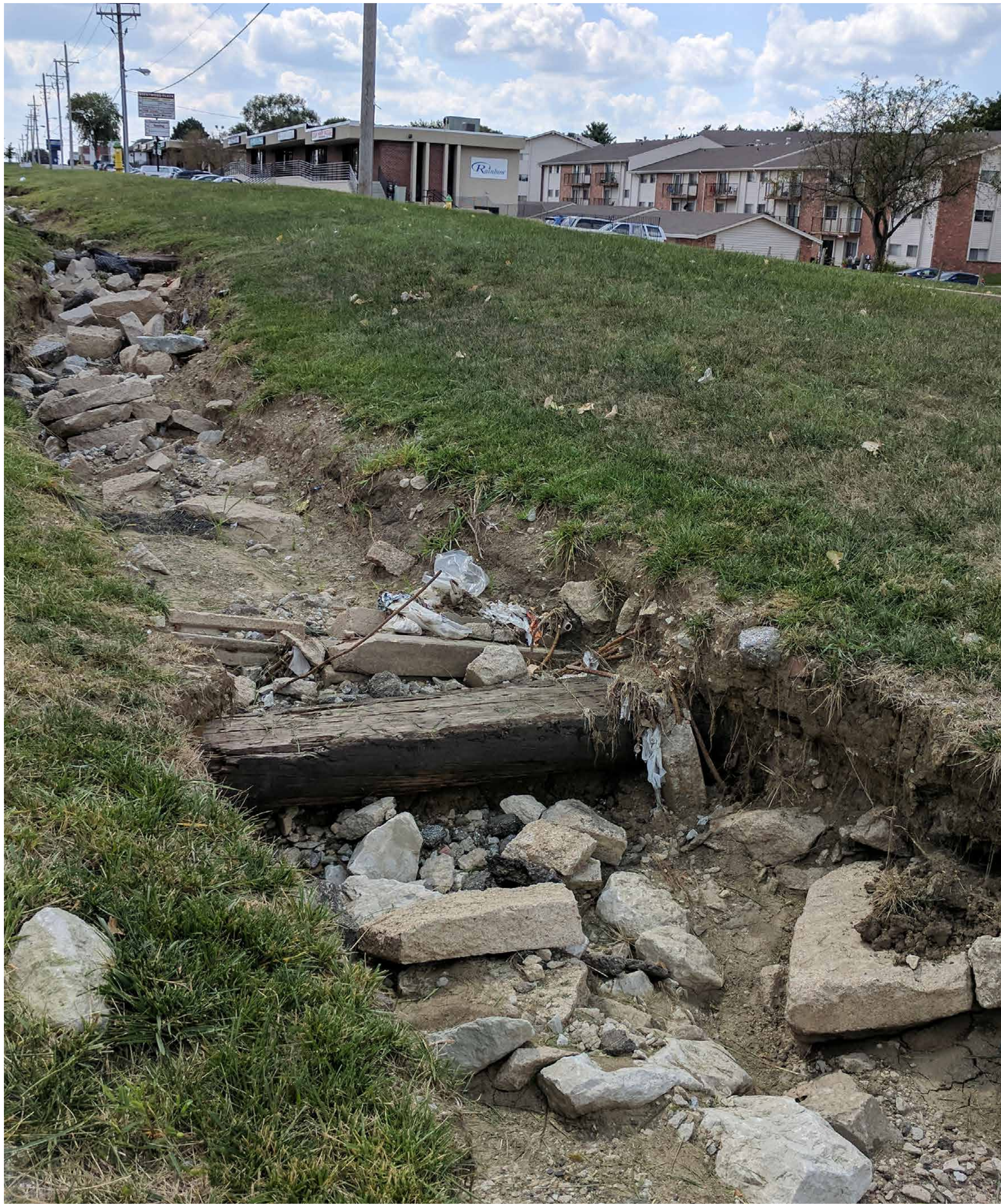
washout in ditch bottom
